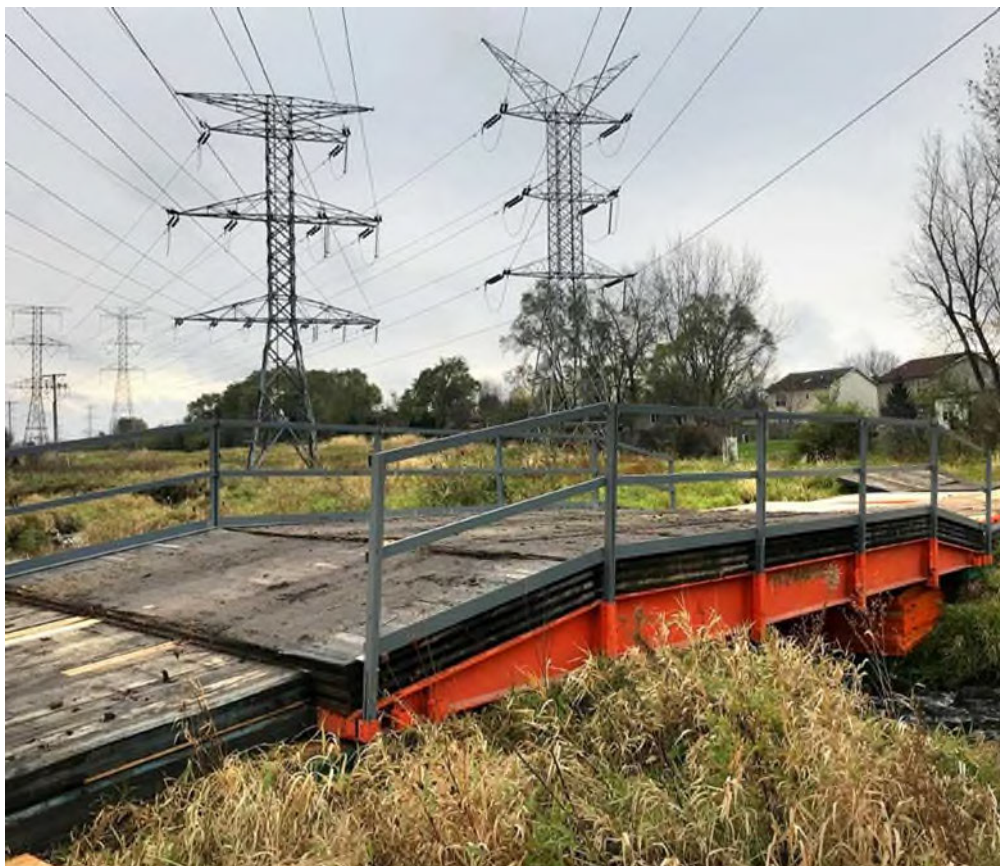
Figure 1.6 – Typical Clear Span Bridge
