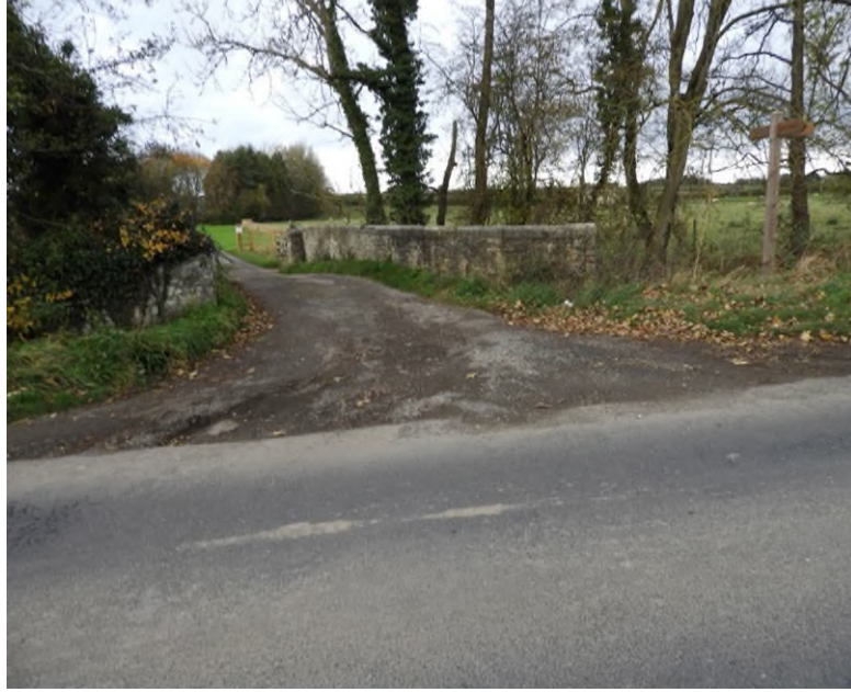
Figure 1.9 – Existing bridge from Wakefield Lane over Cock Beck.
